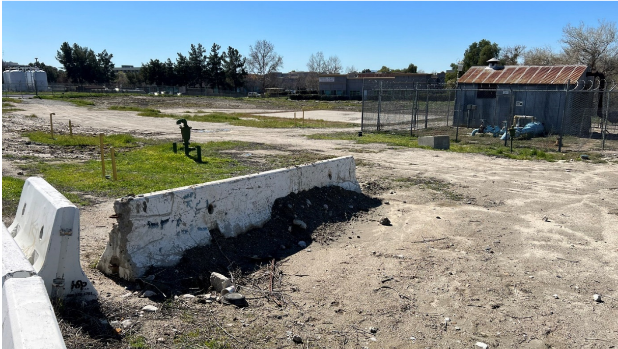
Facing east to adjacent property, possible pump-houses for production wells.
