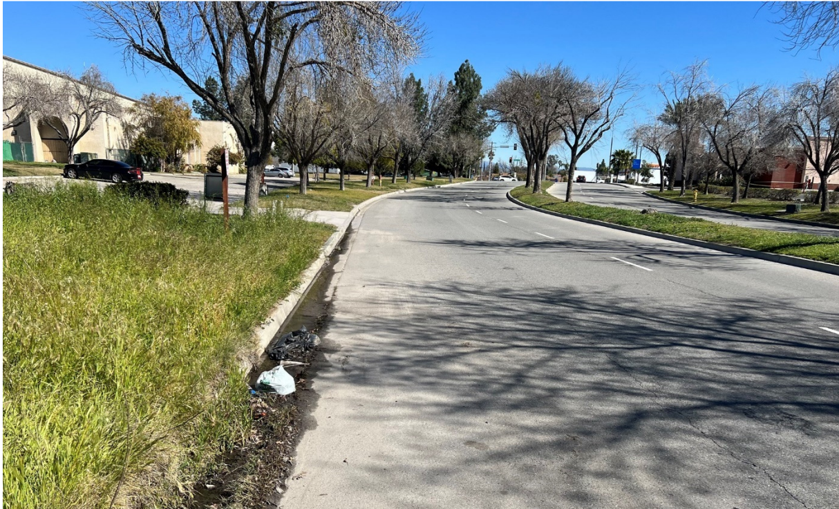
Facing east near subject site southeast corner of the southern boundary along E. Brier Drive.
