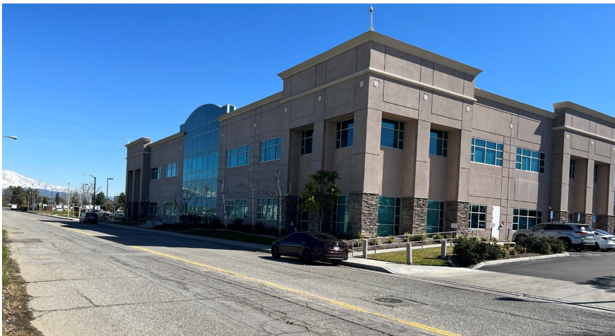
View of adjacent commercial building used by Immigration Services, in between subject site areas, on Hardt Street.
